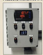
To prevent off-ratio spraying, system will shut down if a pressure imbalance occurs. The system can be easily reset once the imbalance has been resolved.
